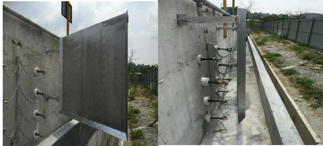
Splash Plate - directs the water from the holes to the drain behind the wall.
